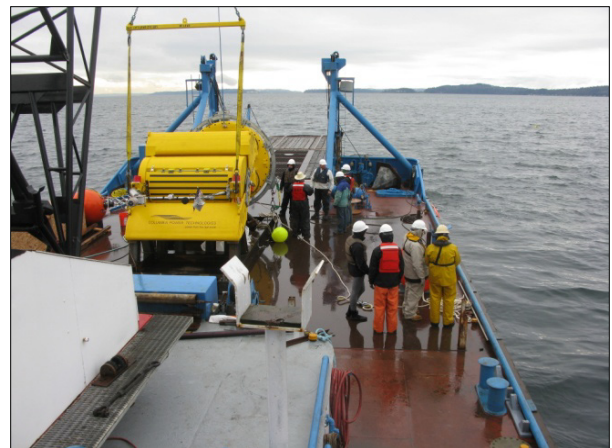
Figure 7 – Sound and Sea Technology helps to install Columbia Power Technologies’ SeaRay wave energy intermediate scale prototype in Puget Sound in 2011.
