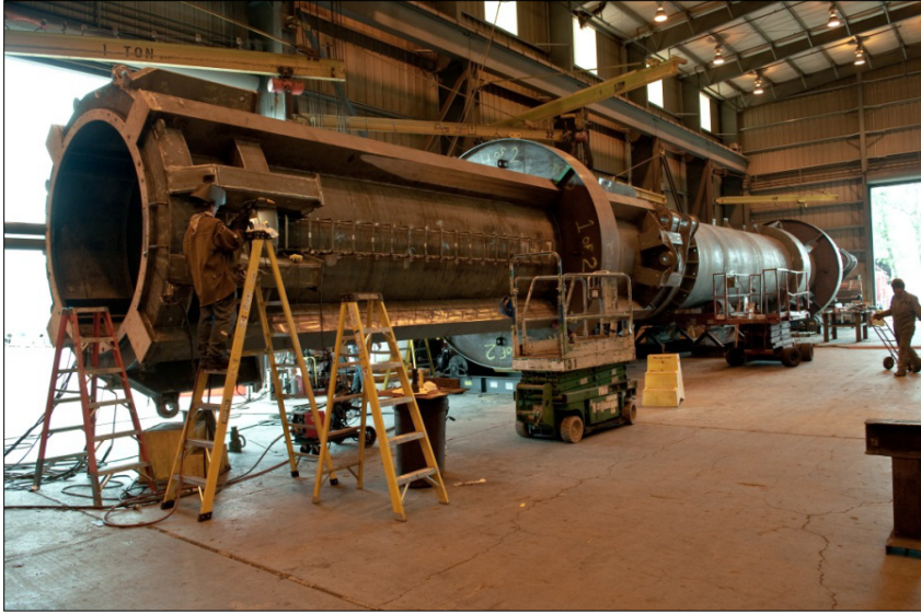
Figure 2 - Part of Ocean Power Technologies' Wave PowerBuoy is assembled at Oregon Iron Works.
